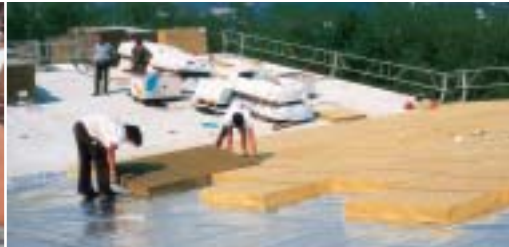
DELTA®-REFLEX PLUS with integrated self-adhesive edge. Typical application on lightweight industrial roof.
