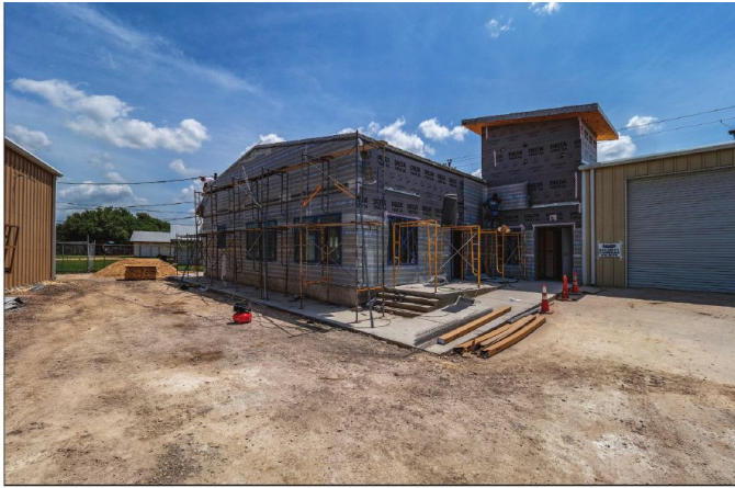
Ventilated rainscreen membrane made of a special high-density polyethylene (HDPE) with pre-installed glass lath.
