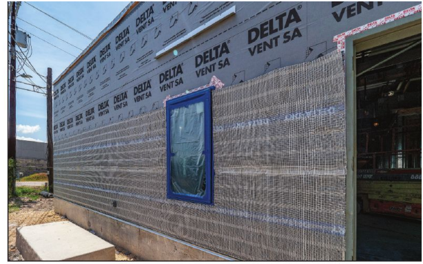
Ventilated rainscreen membrane made of a special high-density polyethylene (HDPE) with pre-installed glass lath.
