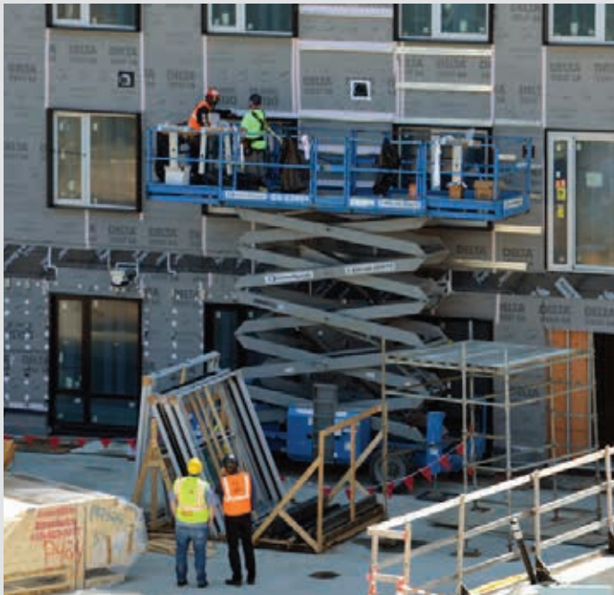
The team installing DELTA®-MULTI BAND 100, a versatile tape with very strong adhesion
