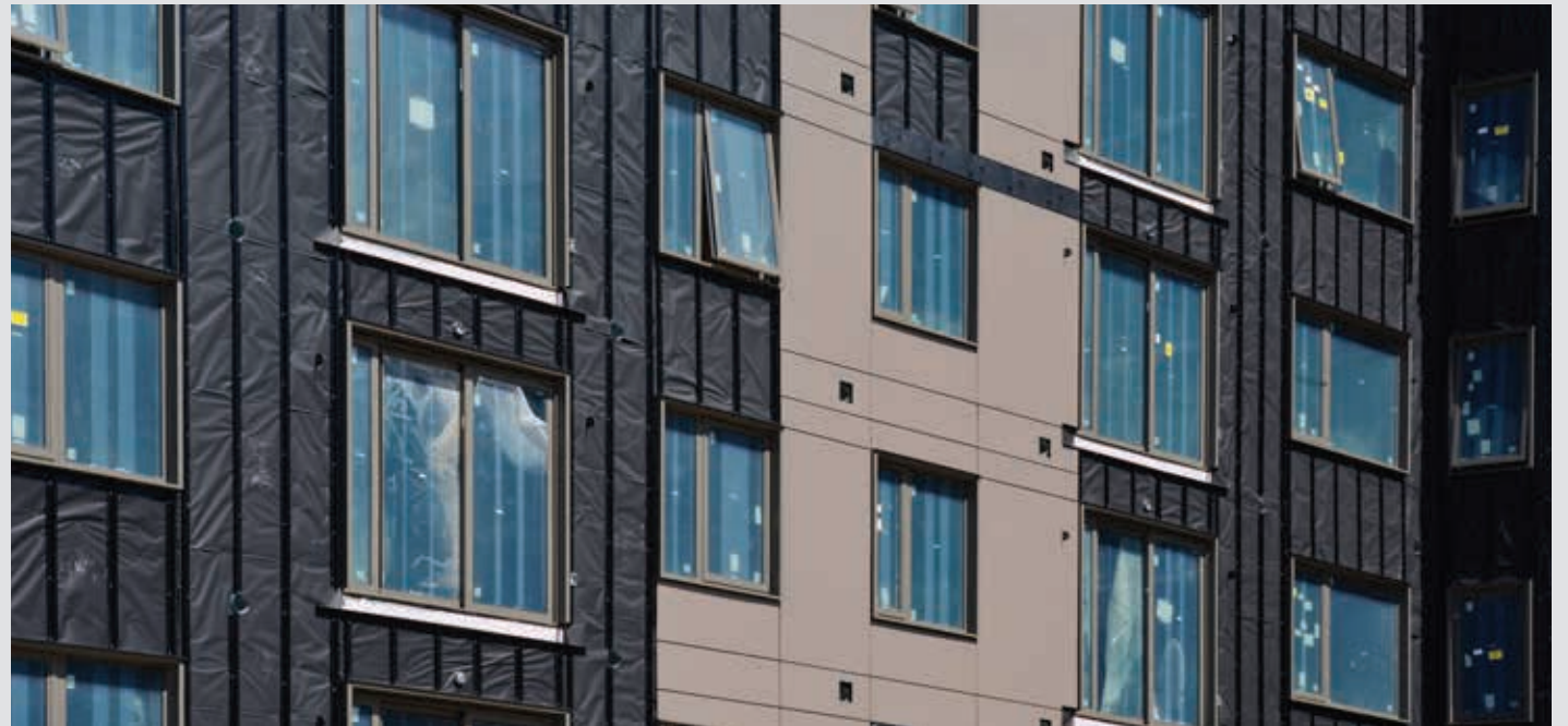
DELTA®-FASSADE S PLUS is highly vapor permeable, and also extremely durable and tear resistant
