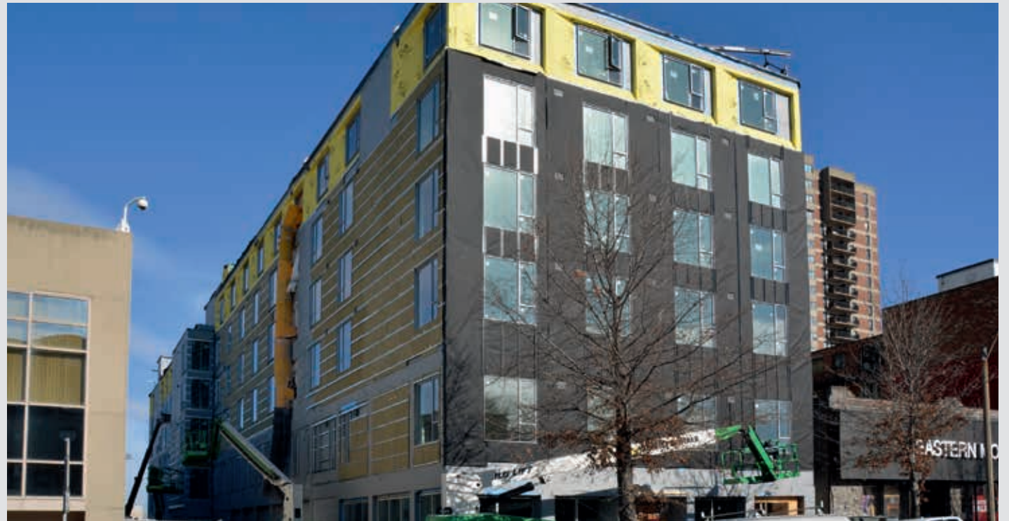
DELTA®-FASSADE S is designed specifically for the demands of open-joint cladding
