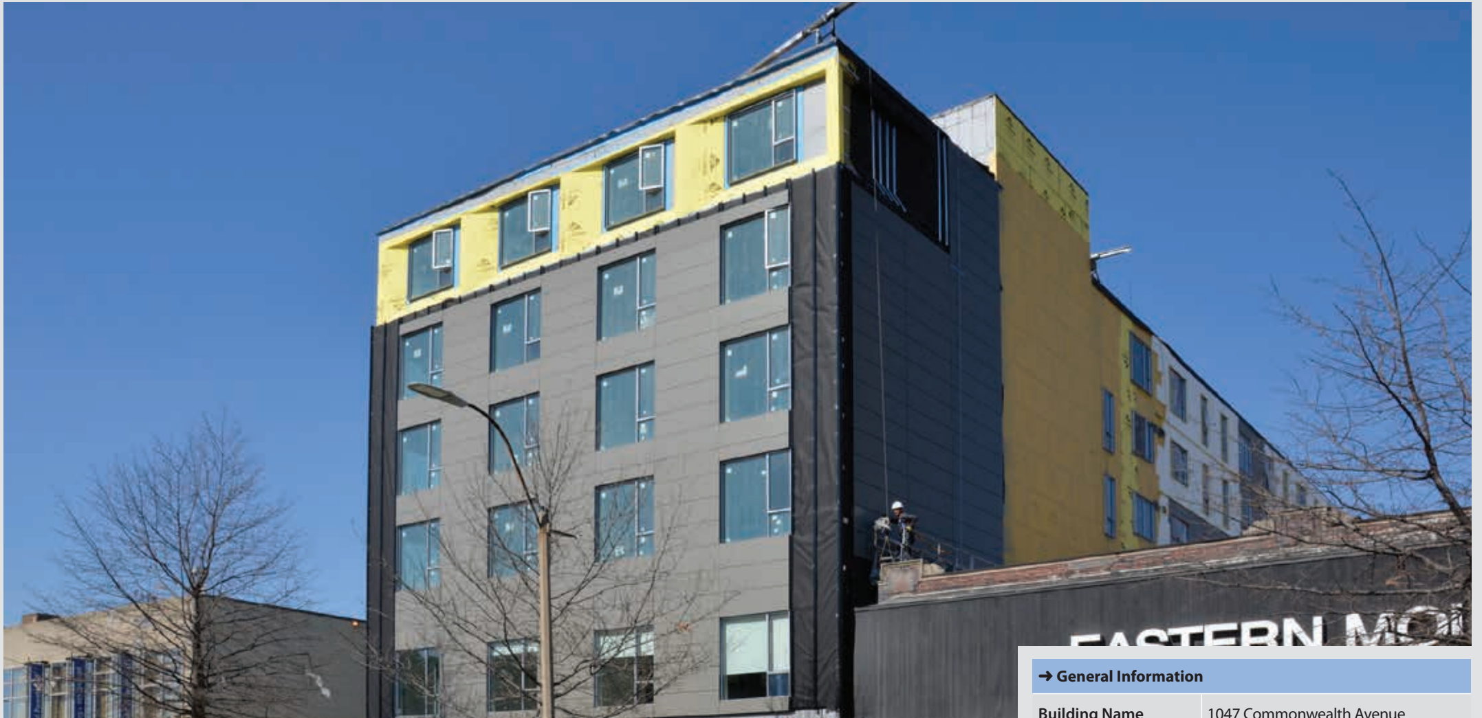
1047 Commonwealth Avenue, originally a two-story building, was expanded to six stories to create 180 studio apartments
