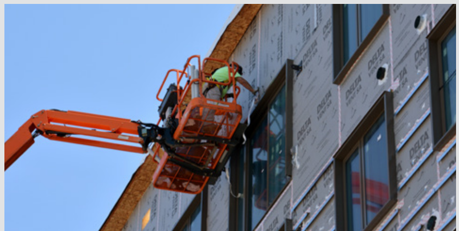
DELTA®-VENT SA is a vapor permeable air- and water-resistive barrier that prevents moisture from getting into buildings
