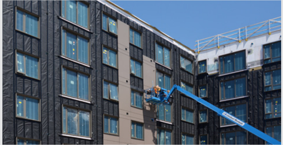
DELTA®-FASSADE S PLUS is highly vapor permeable, and also extremely durable and tear resistant
